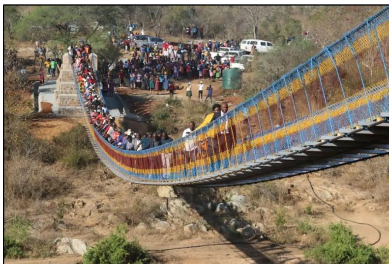
Picture 3: Inauguration of Mankantimane Suspended Foot Bridge at Luhlanyeni Chiefdom under Sithobela Constituency.
