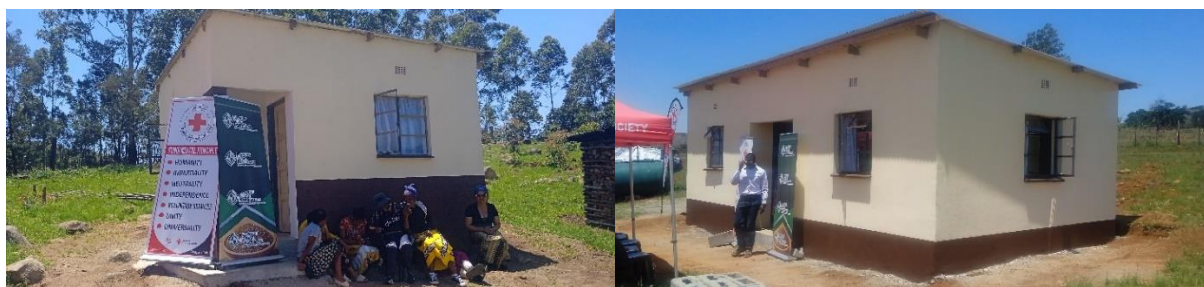
Picture 7: Newly constructed one room house for the elderly at Mnyokane and a two-room house for OVC at Motjane
