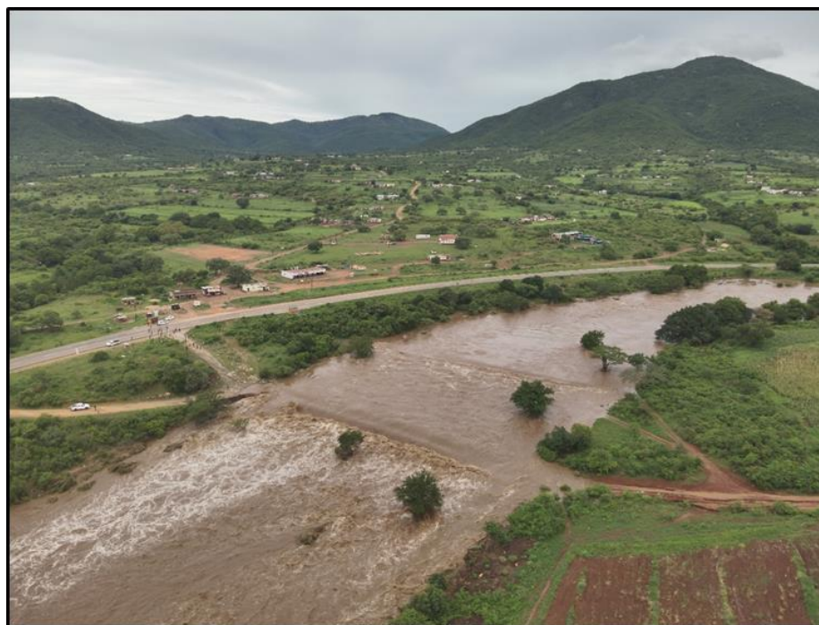
Picture 1: A low laying bridge in Nkhwe Community under Nkwene Inkhundla completely submerged as a result of 6-8 January 2025 Torrential rains.
