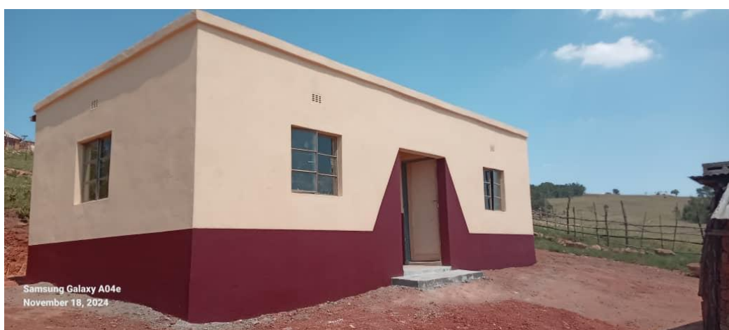
Picture 8: Two-room house handed over at Dudusini, Ngwempisi Constituency
